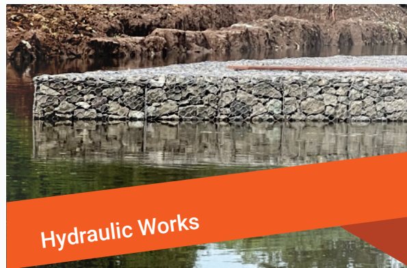
Coastal & Pipeline Protection
